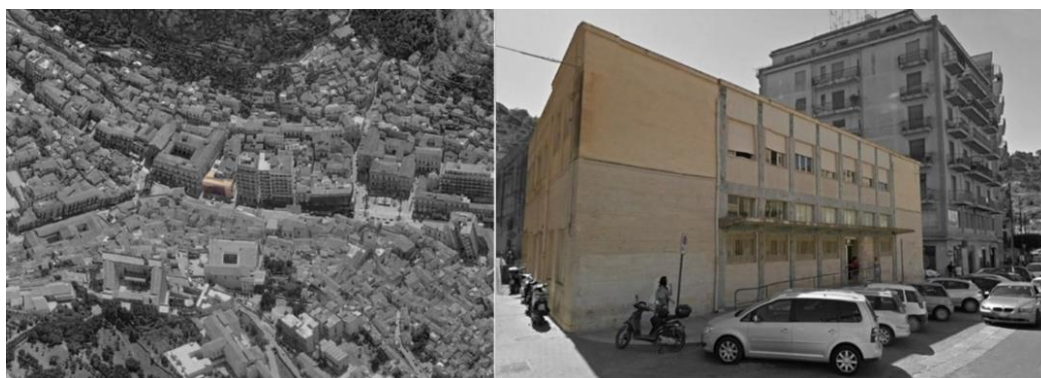
Figure 1. Former Post Building.
