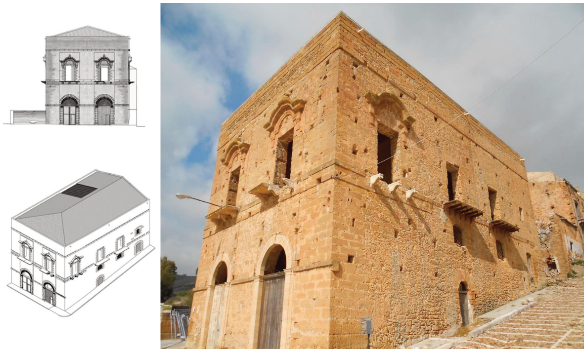
Figure 4. Restoration of representative buildings: Palazzo Tamburello-Agosta (Museum of Popolar Traditions).
