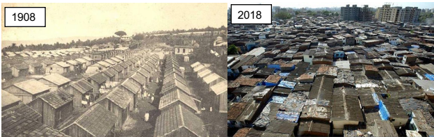
Fig.1: Temporary housing in Messina (Sicily)
