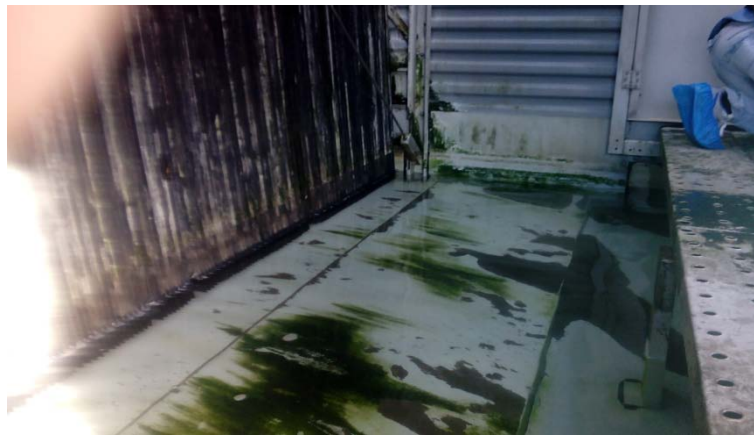
Photograph 2 : Visual inspection of the collecting basin - November 2014
