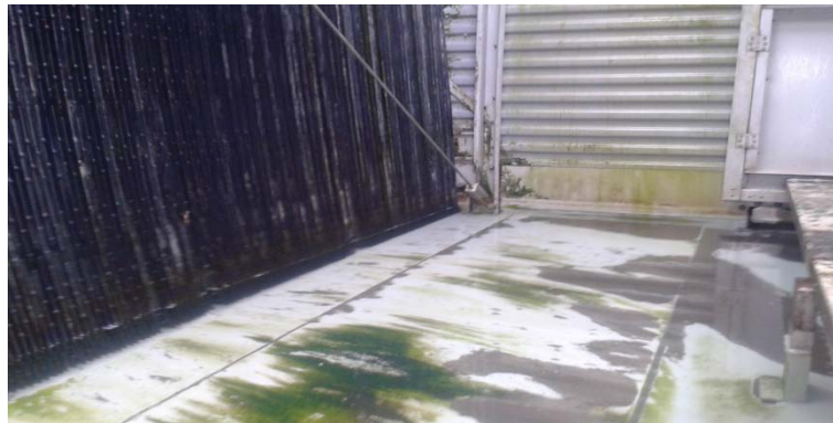
Photograph 3 : Visual inspection of the collecting basin - January 2015
