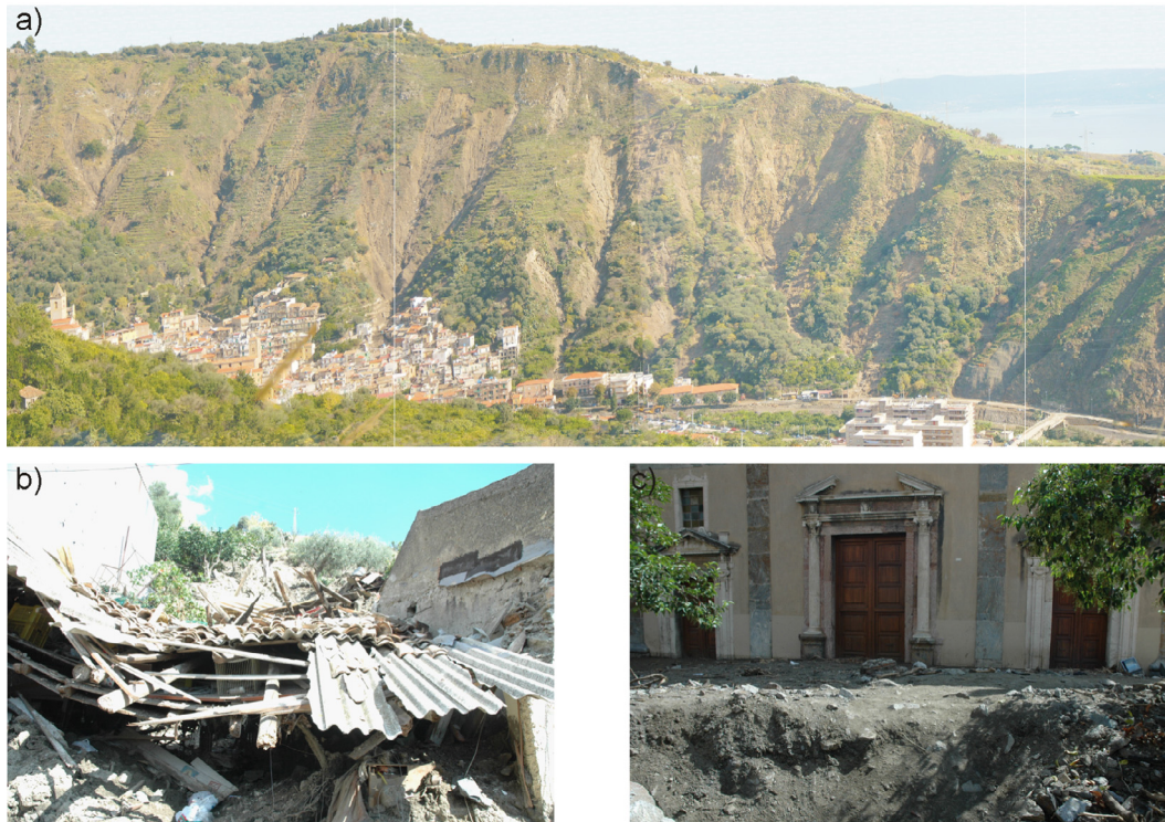
Fig. 5. Photo-panorama of Giampilieri village after the alluvial event: a) the slope scoured by debris flows; b) Giampilieri urbanized area damaged by the alluvial event; c) Giampilieri urbanized area where the sediment deposit level is recognizable.
