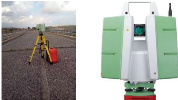
Fig.3. Terrestrial Laser Scanning TLS survey during the bridge monitoring.
