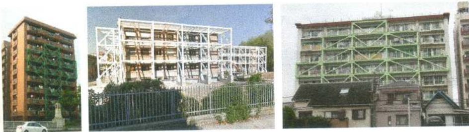
Figure 3. Examples of seismic retrofitting with steel exoskeletons.
