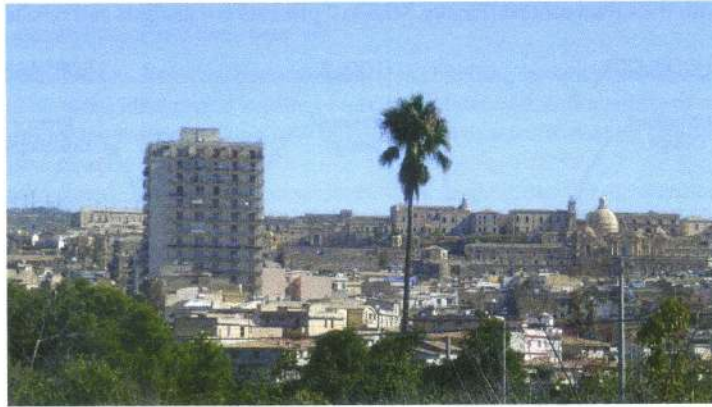
Figure 1. An example of a reinforced concrete building that does not take into account the aesthetic value of its urban landscape nor the seismic risk of the area in the Baroque city of Noto, Italy.
