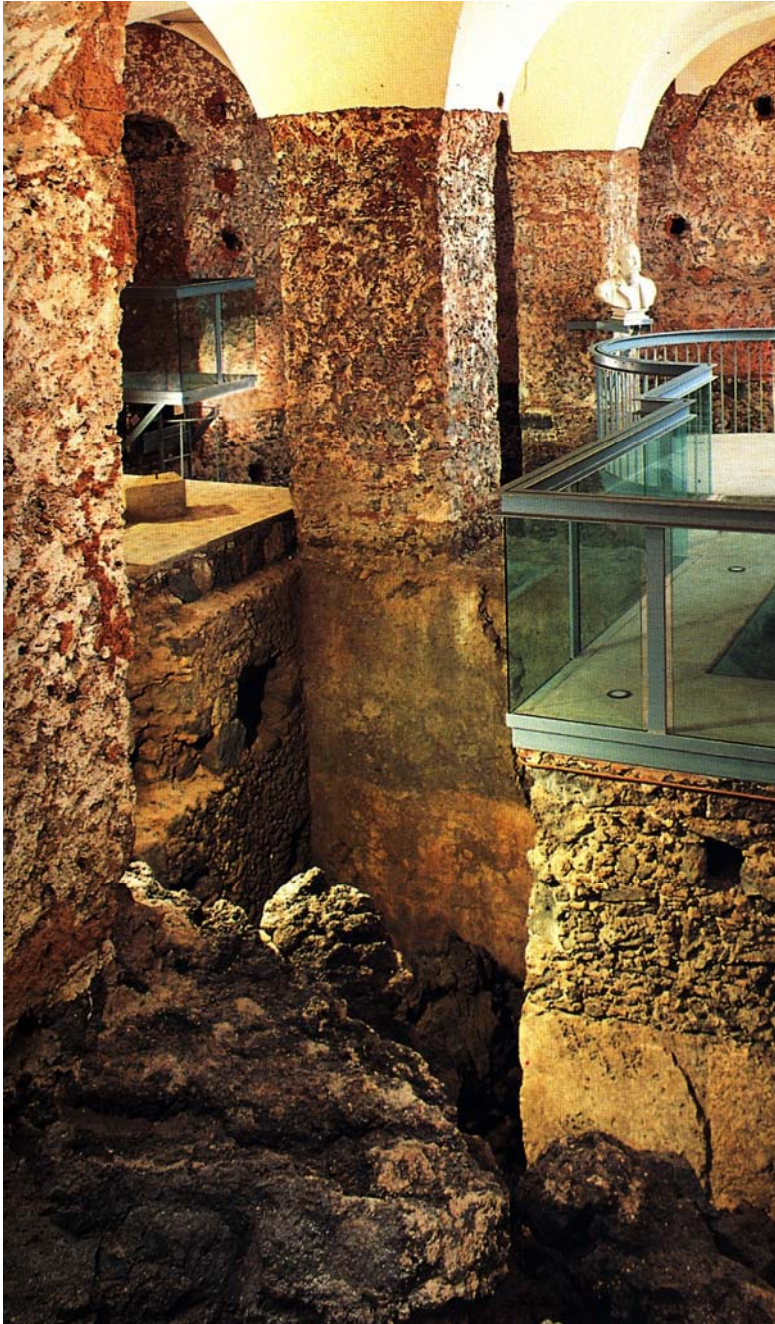
Fig. 3 - Rooms on the lower floor previously used by the Geodynamics Laboratory, in the foreground the 1669 lavaflow © F.M.C. Santagati
