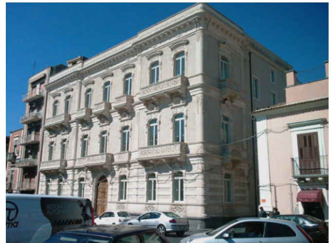
Fig. 8. Restoration site where the mortar was used – “Palazzo Porto” Catania.
