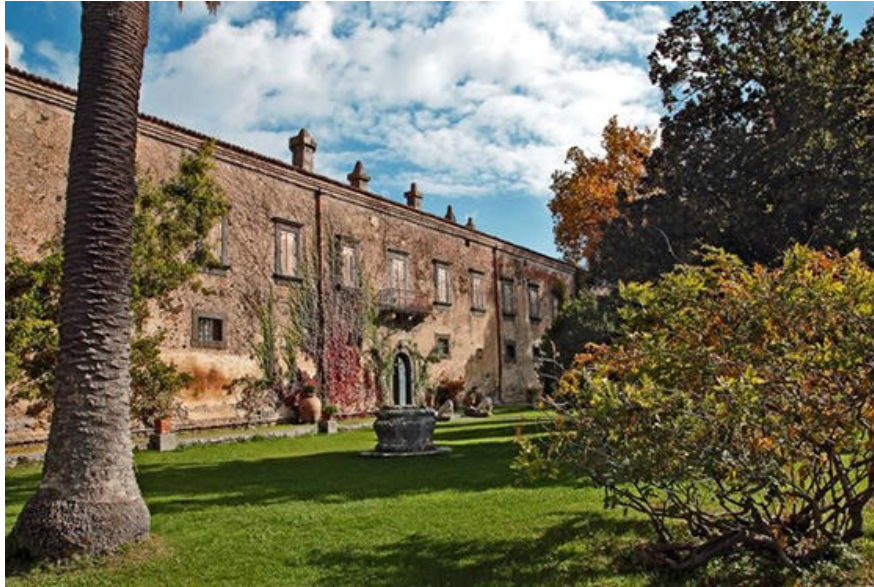
Fig. 1. The Nelson's Castle, which involves the reuse of recycled aggregates from the same restoration site.
