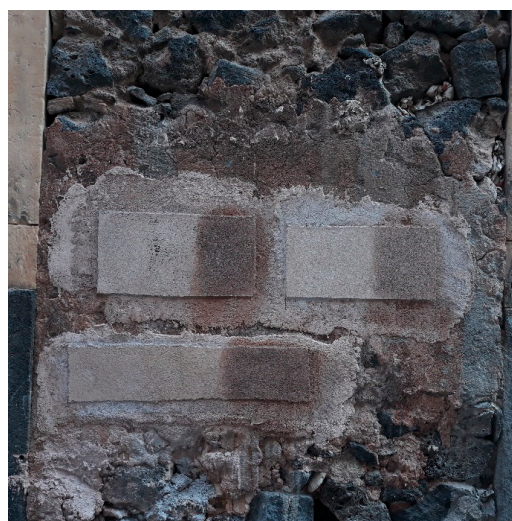
Figure 11. Some tests on different mix design and finishing (photo by Lo Faro A).
