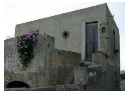
Figure 3. Two-cell house (horizontal type)
