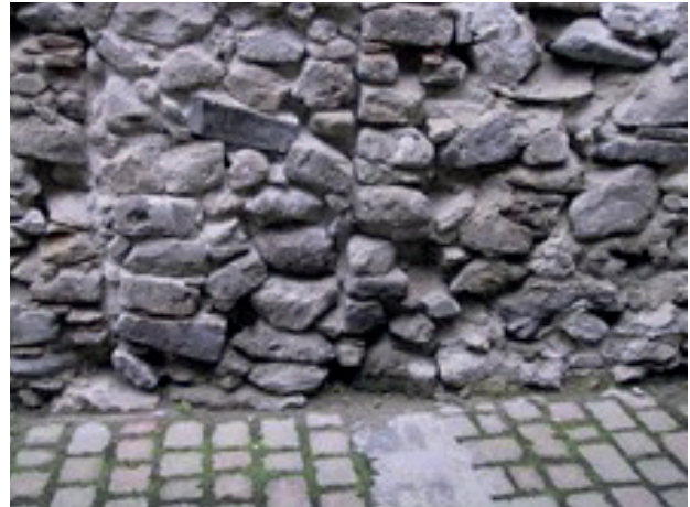
Figure 10. Shapeless stones wall
