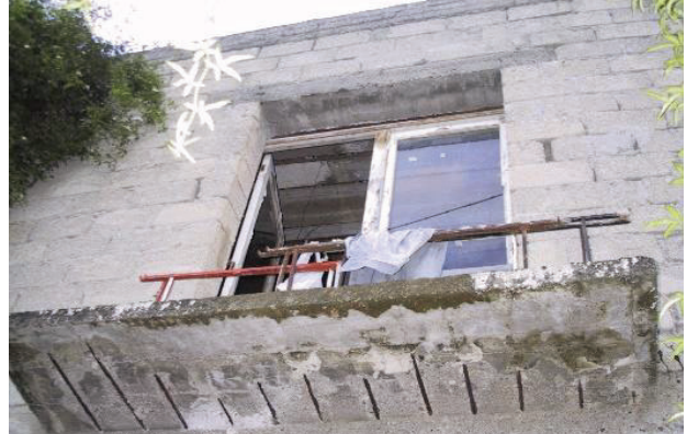
Prefabricated joists and hollow clay blocks floor
