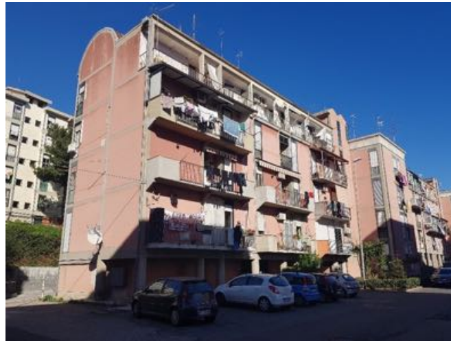
Figure 6. Multi-story apartment building selected as the case study.
