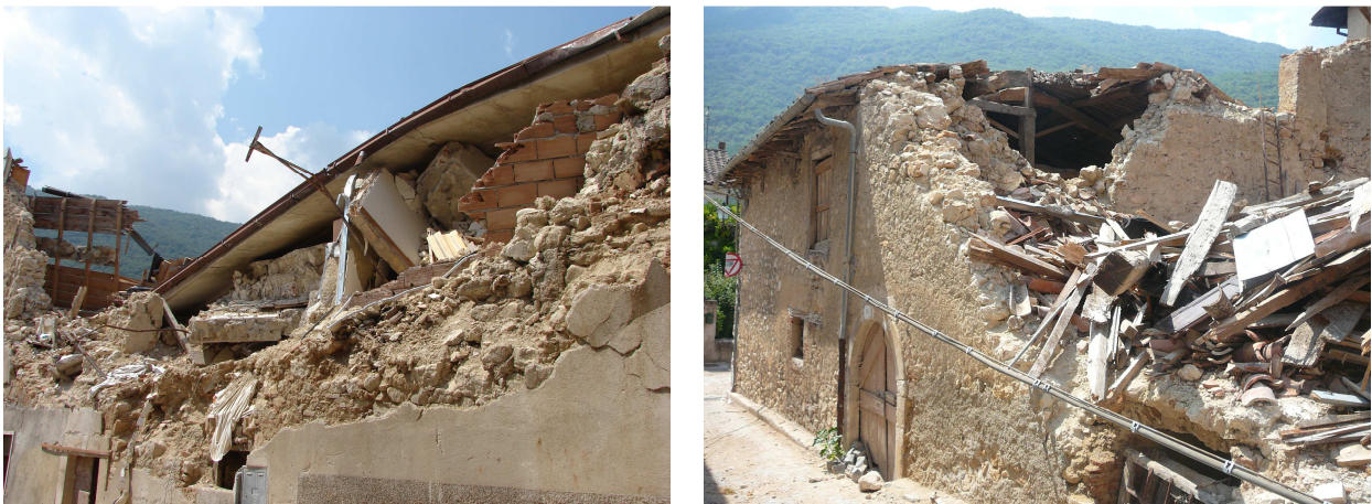
Figure 4: Vulnerability (heavy r.c. roof structure) and resistance (anchored trusses) factors
