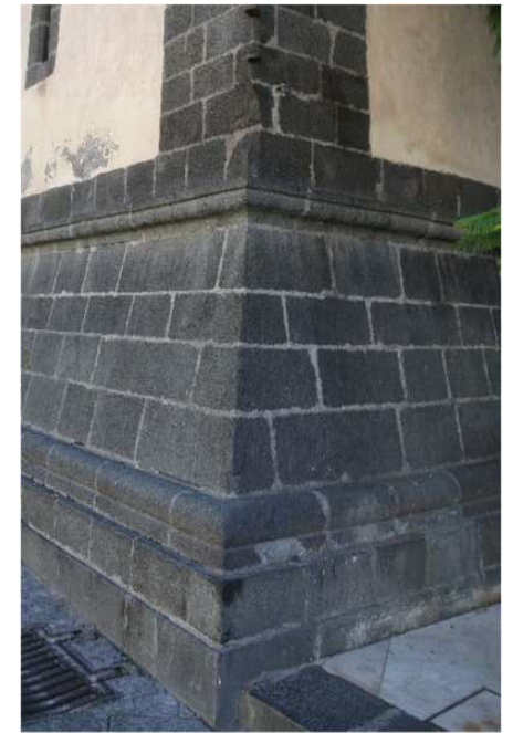
Figure 4. Scarp base with basalt canmarozzoni in the south bell tower of the Mother Church of Acireale (photo: L.P. Alfonso).
