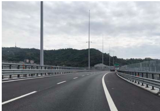
Fig. 2. Genoa Bridge pavement (2021)
