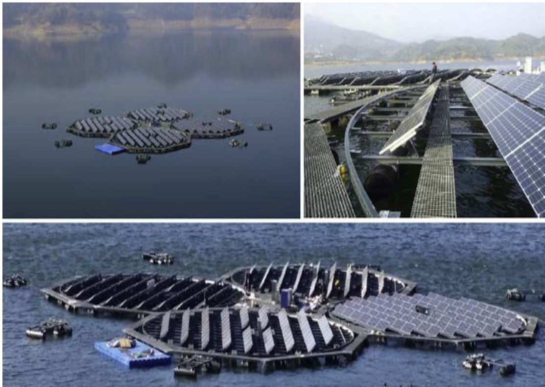
Figure 18 K-water tracking installation
