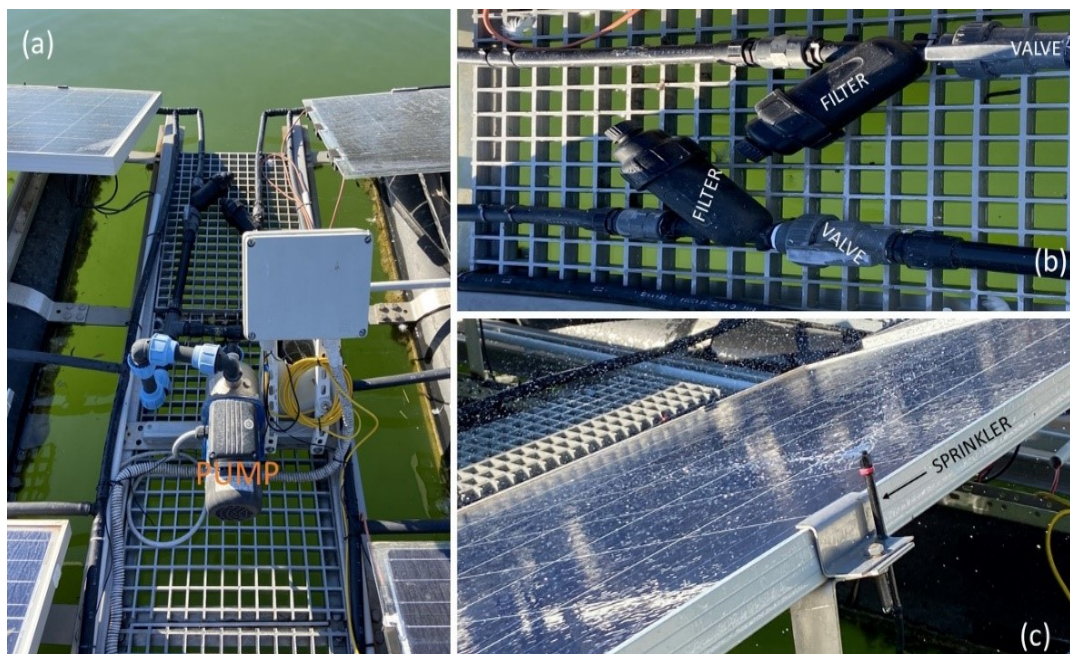
Figure 27 Components of cooling system
