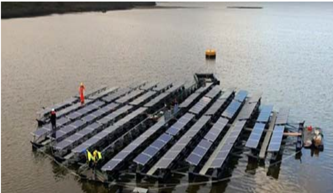
Figure 16 Rope system which allows 2 or 1 axis tracking
