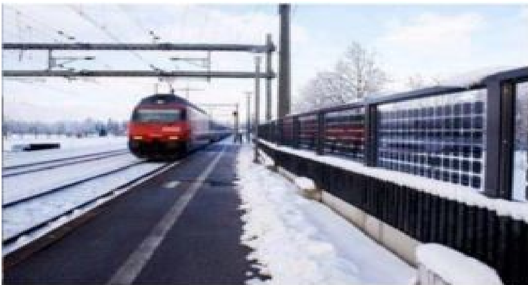
Figure 9 Noise barriers with bPV [21]
