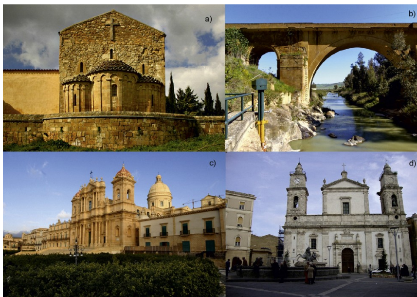
Figure 1.4 - The use of Sabucina Stone in some representative monuments of southern Italy. (a) S. Spirito Church; Caltanissetta (1151); (b) Capodarso bridge (1556); (c) Noto Cathedral (1703-2007); (d) Caltanissetta Cathedral.
