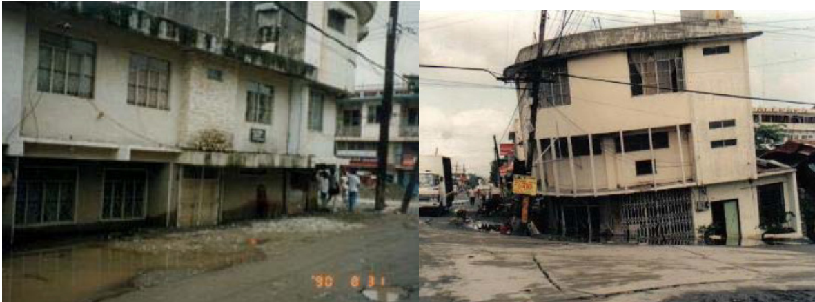
Figure 2.12 Settlements and tilting of buildings following the 1990 Luzon earthquake (From Orense, 2011).
