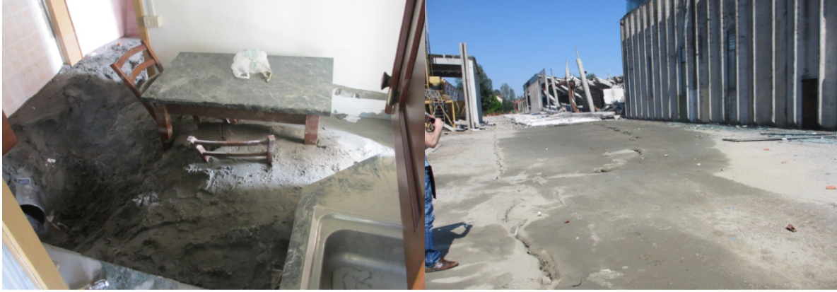
Figure 2.16 Liquefaction evidences observed immediately after the earthquake (From Vannucchi et al., 2012).
