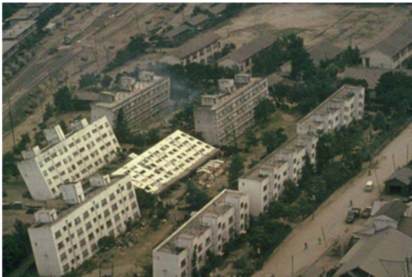
Figure 2.11 Liquefaction-induced bearing capacity failures of the Kawagishi-cho apartment buildings following the 1964 Niigata earthquake (From Kramer, 1996).
